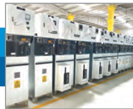
MODULAR ENCLOSED SWITCHEGARS (up to 12, 24, 36, 40,5kV 25kA)
