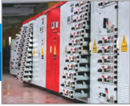
LV PANELS (from TEDAŞ switchboards type 4b-withdrawable, up to 6400A-100kA)
